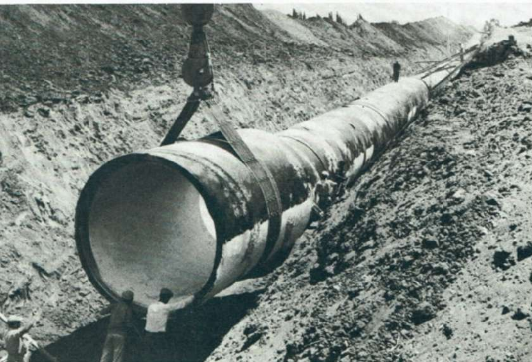
LAYING THE 108" PIPES
